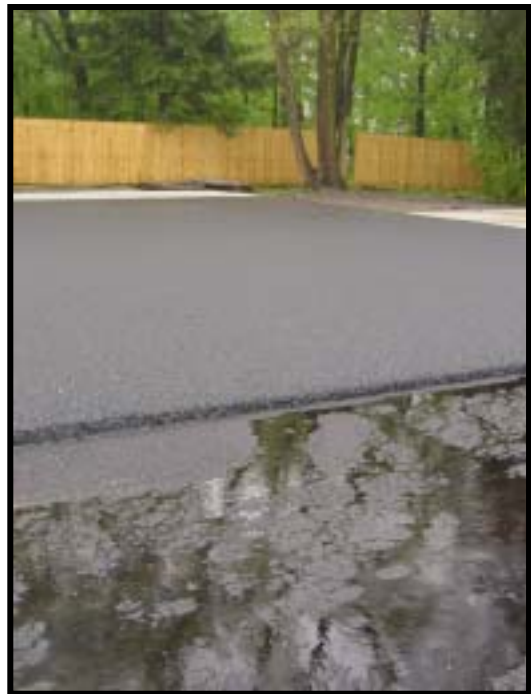
Pervious asphalt paving
